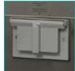
Duplex and/or GFI Outlets
